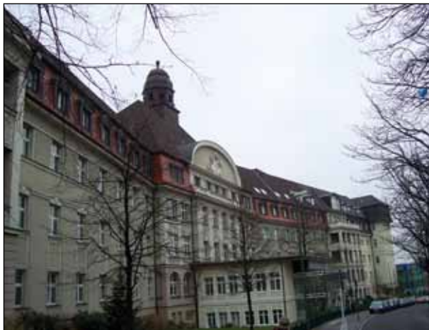
The Elizabeth Krankenhaus in the Contilia group houses nearly half of the total of three hundred cardiac beds in the group. The hospital is currently installing a new CVIS PACS system connecting processes and images of Cath Lab, ECG, Echo, EP-Lab, Cardio-Surgery and Cardio Visit. .
